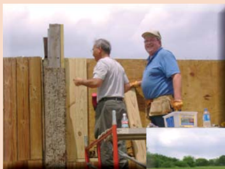
Hoa Nguyen and Van Elliott putting up new baffle boards
