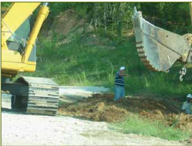
TRA construction being directed by Ken English
