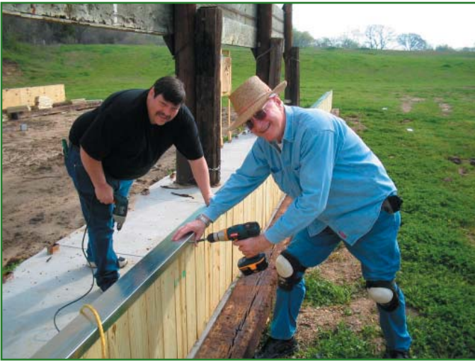
David Anderson & Kerry Williams installing rain caps
