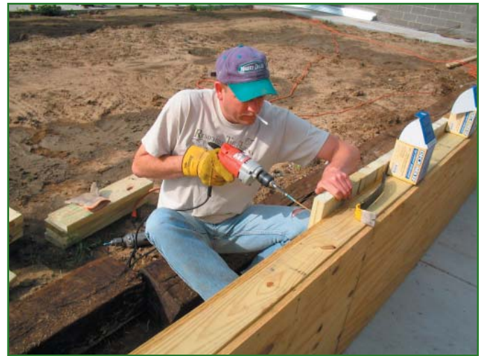
Forrest Weaver placing 2x6 facings
