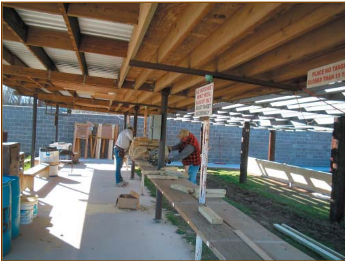
bill Schweitzer & Terry Cullender cutting and pre-drilling
