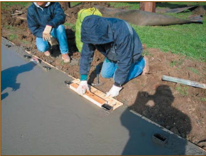
Aligning the target frame sleeves
