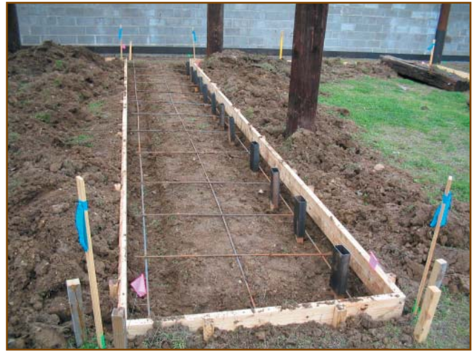
Pistol range sidewalk and target line formed (new 7-yd. line)
