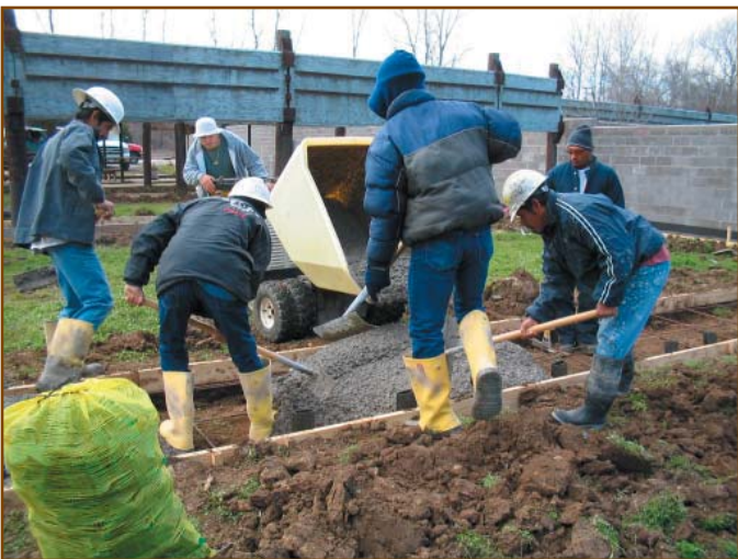
Here comes the concrete
