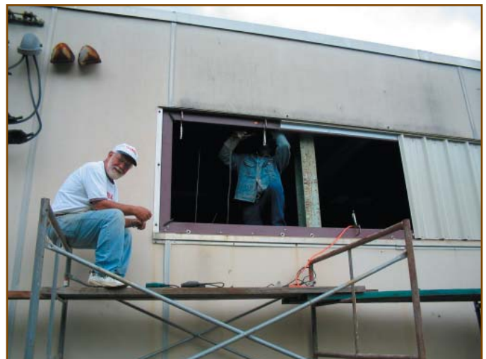
Ken English watching Steve Gilmore welding
