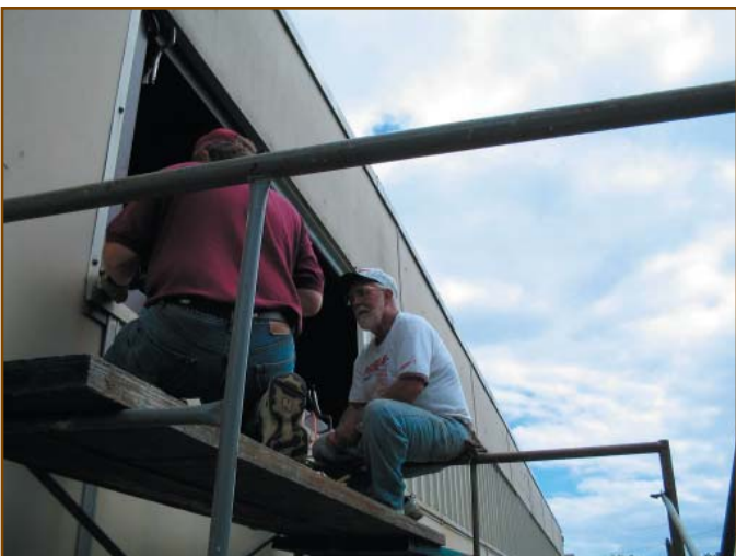
Randy & Ken replacing metal on the old building
