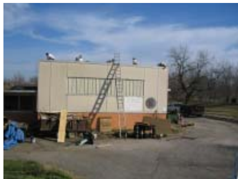
Roofing the shop
