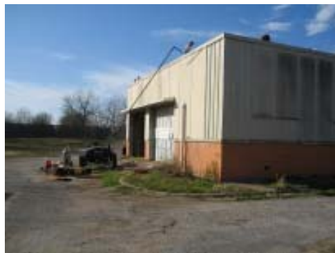
Reroofing the shop
