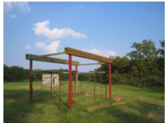
Skeet Field #5 under construction
