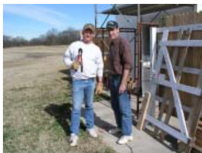
Bill Schweitzer & Jeff Zwiebel rebuilding fence and building fascia
